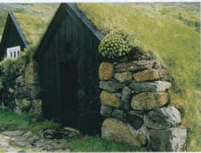
Early Icelandic structures featured roofs of sod and turf (top, above), which have become hallmarks of Icelandic vernacular architecture.
