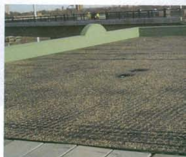
As rendered in this computer-generated image (top), the green roof planned for PEEC will replace asphalt (above) with plants for storm-water retention and seating areas for employees.
