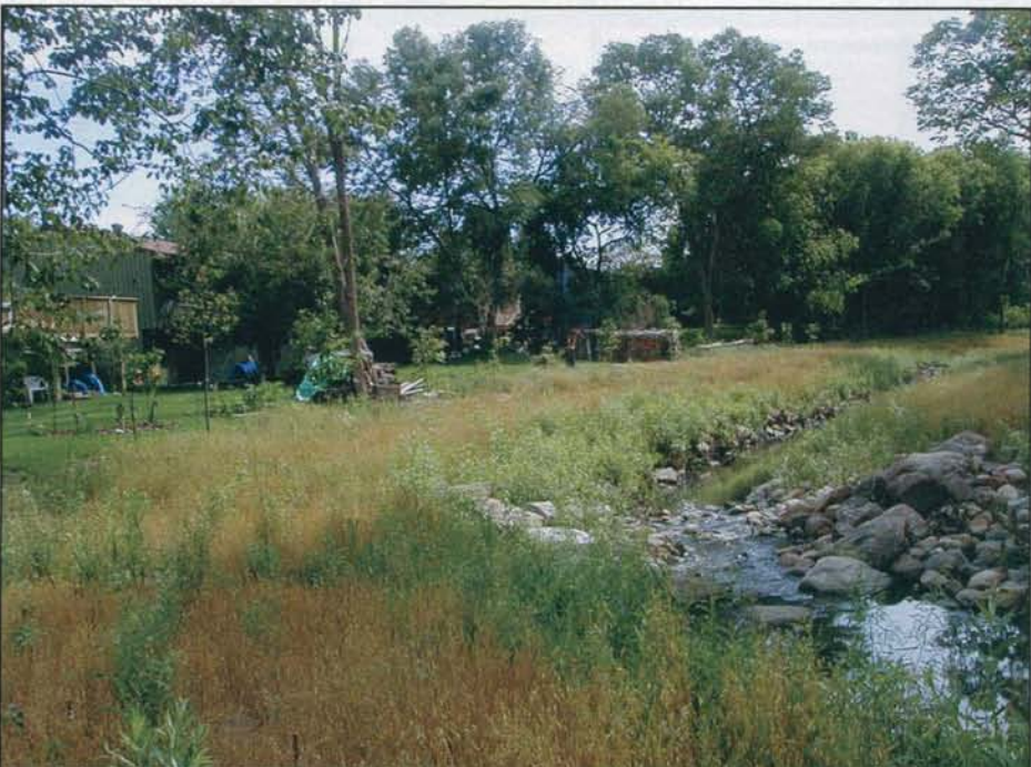
After: The community-endorsed design solution used native vegetation and soil bioengineering techniques to restore the Pike Channel to an open canopy, savanna/prairie plant community that is now a community asset.
